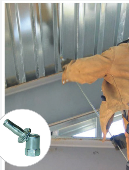
SXP 20 Installation Fort Bragg, N.C., construction
